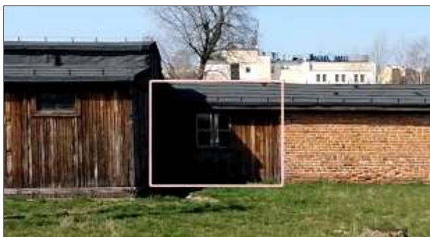
Left: bath and disinfection building no. 1 at Majdanek Camp. Right: disinfestation building containing Rooms I-III. In a white box: structure fraudulently added after the war connecting the two buildings.
